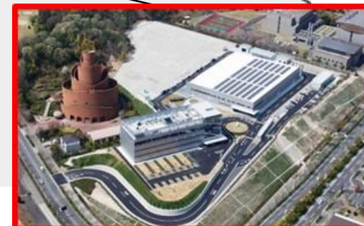
Technical Center Kizugawa Works
